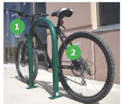
Image 14: Two points of contact reduce the possibility of tipping.
