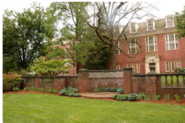
The brick and cast stone terrace wall, designed by Ellis Lawrence and constructed in the 1920s.
