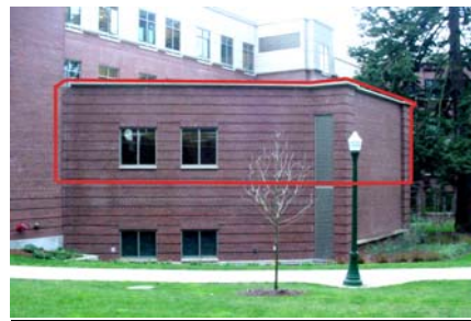
Fig. 2: Northwest facade of Room 282. Stack air inlets visible at right and operable windows at left.
